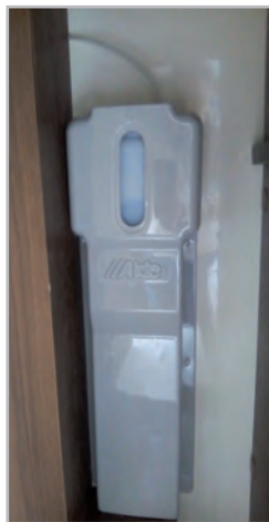
Fig.6.41 - Glycol mixture level
