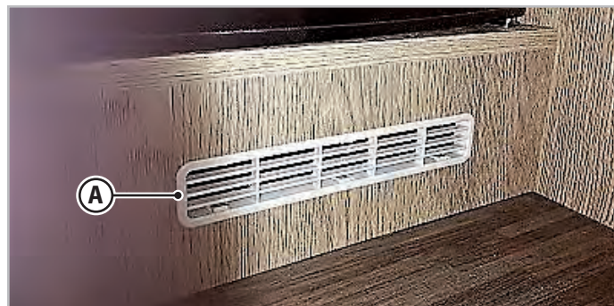
Fig.6.1 - Permanent ventilation openings
